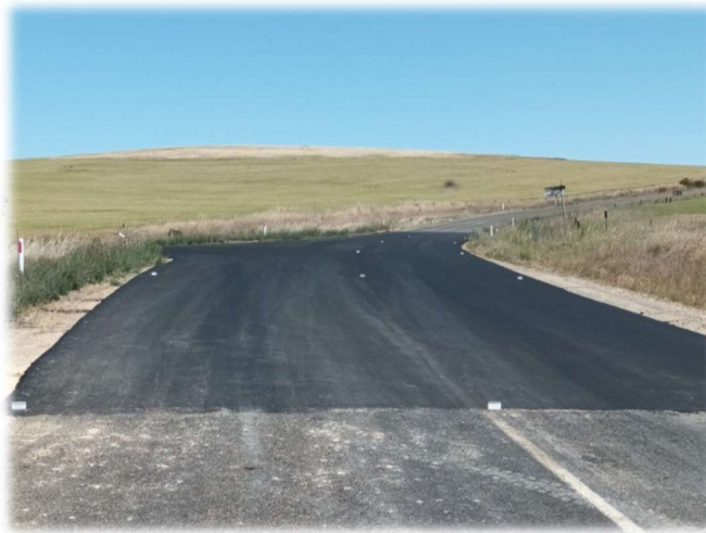
Gum Creek Rd intersection sealing
