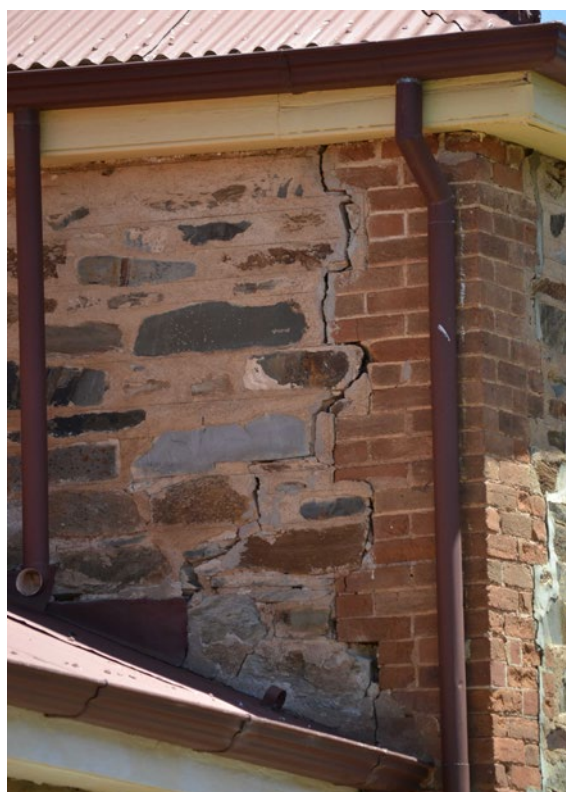
Redruth Courthouse (SAHR 10027) (Currently not mentioned in the National Heritage Values) – Cracking to corner
