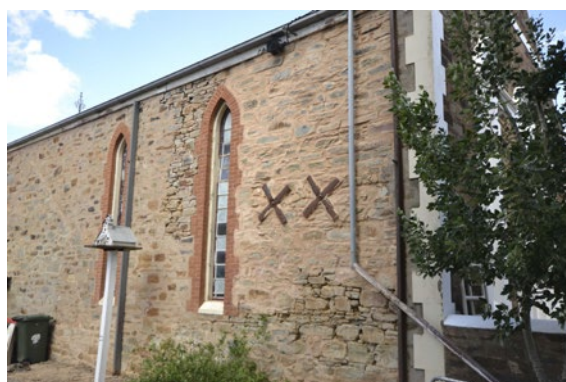
Kooringa Primitive Methodist Church (10011) – Deterioration of mortar joints to upper walls caused by blocked or leaking gutter
