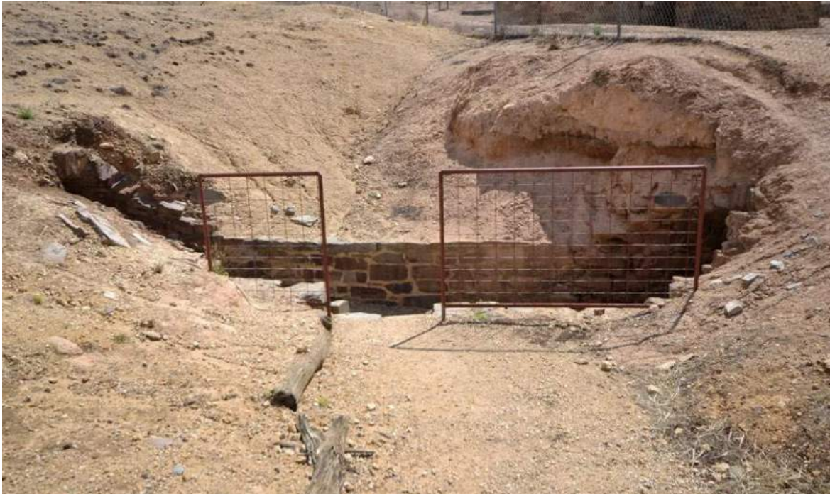
Open Section of Flue between Boiler House and Chimney
