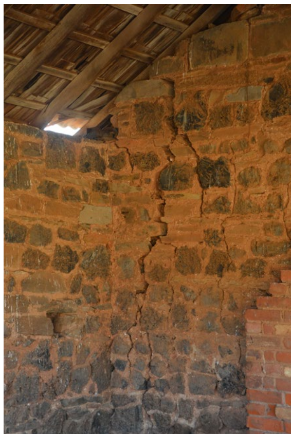
Smeltsyard (SAHR 10024) – Major cracking
