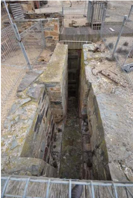
Balance Beam Slot
