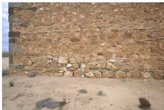
Powder Magazine (SAHR 10045) – Deterioration of mortar at base of walls
