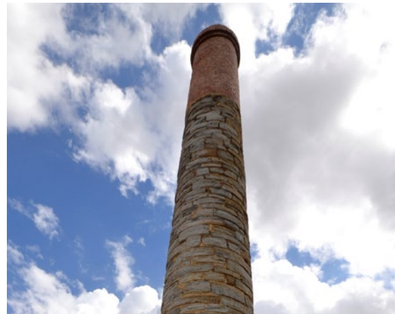
Cornish Crusher Chimney/Dressing Tower Complex (SAHR 10047) – Deterioration of pointing and stone surfaces to leeward side
