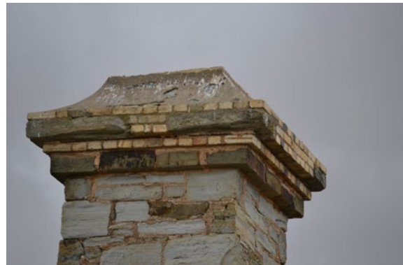
Haulage Engine Chimney (SAHR 10046) – Horizontal gap at the bottom of the chimney coping likely caused by oxide jacking
