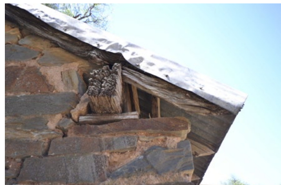
Redruth Courthouse (SAHR 10027) (Currently not mentioned in the National Heritage Values) – Weathering to end of timber wall plate and end of rafter/barge to outbuilding
