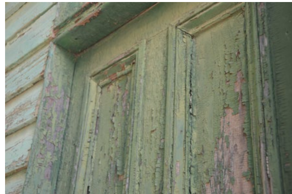
1840s Timber Dwelling (SAHR 10434) – Failure of paint finish to door leading to weathering of timber substrate
