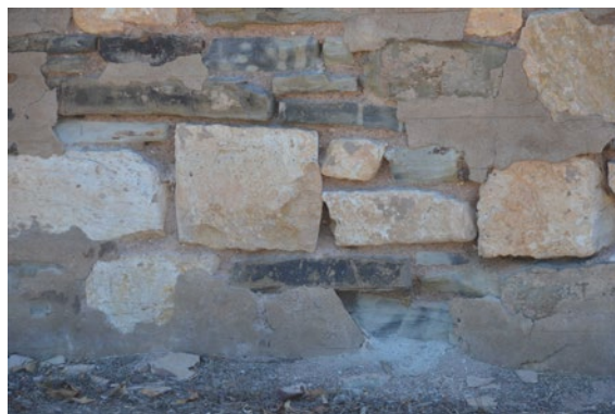
SAMA Yard and Walls (10019) – Deterioration of mortar and stone at base of east wall
