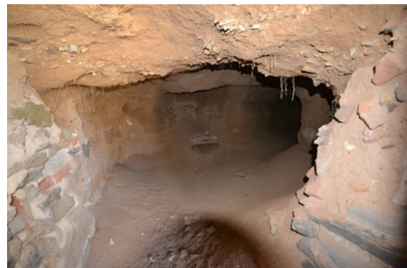
Miner's Dugouts (SAHR 10050) – Deterioration of clay ceiling and wall surfaces
