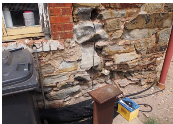
Former Mine Hospital (Currently not mentioned in the National Heritage Values) – Significant deterioration of stone probably due to internal moisture issues associated with services and concrete floor
