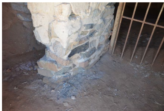
Miners Dugouts (SAHR 10050) – Deteriorated stone to base of walls
