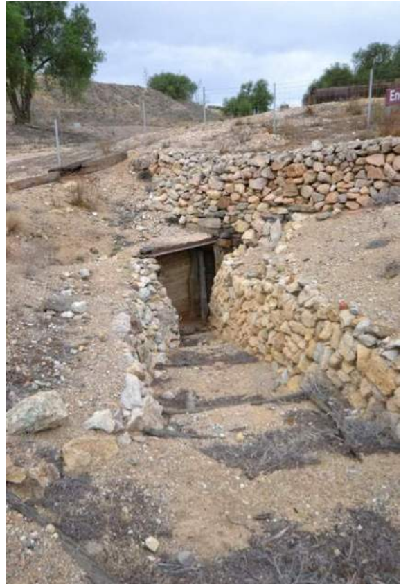
Opening in side of Drainage Adit
