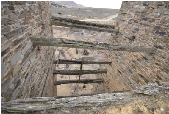
Former Engine/Crusher house (SAHR 10445) – Deterioration of remaining timber beams bracing external walls
