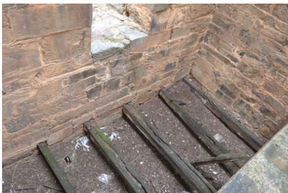
Graves Pump House (SAHR 10054) – Deterioration to timber joists within cockpit
