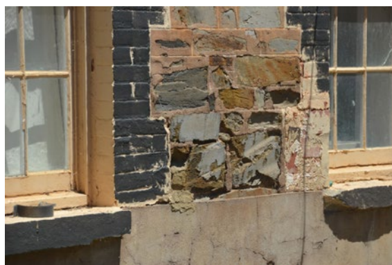
Burra Hotel (SAHR 10404) – Deterioration of stone over cement render repair to lower portion of wall
