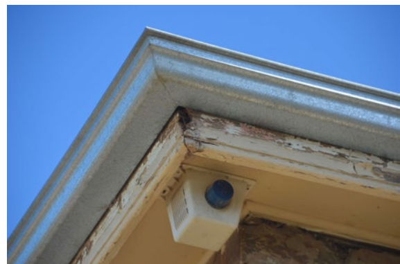
Burra Town Hall (SAHR 10403) - Deteriorated paint finish to fascia leading to weathering of timber substrate
