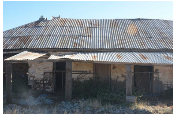
Smeltsyard (SAHR 10024) – Missing roof sheeting and flashings
