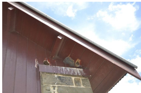
Morphett's Enginehouse (SAHR 10053) – Holes made by starlings through timber linings to access nesting sites within the roof void
