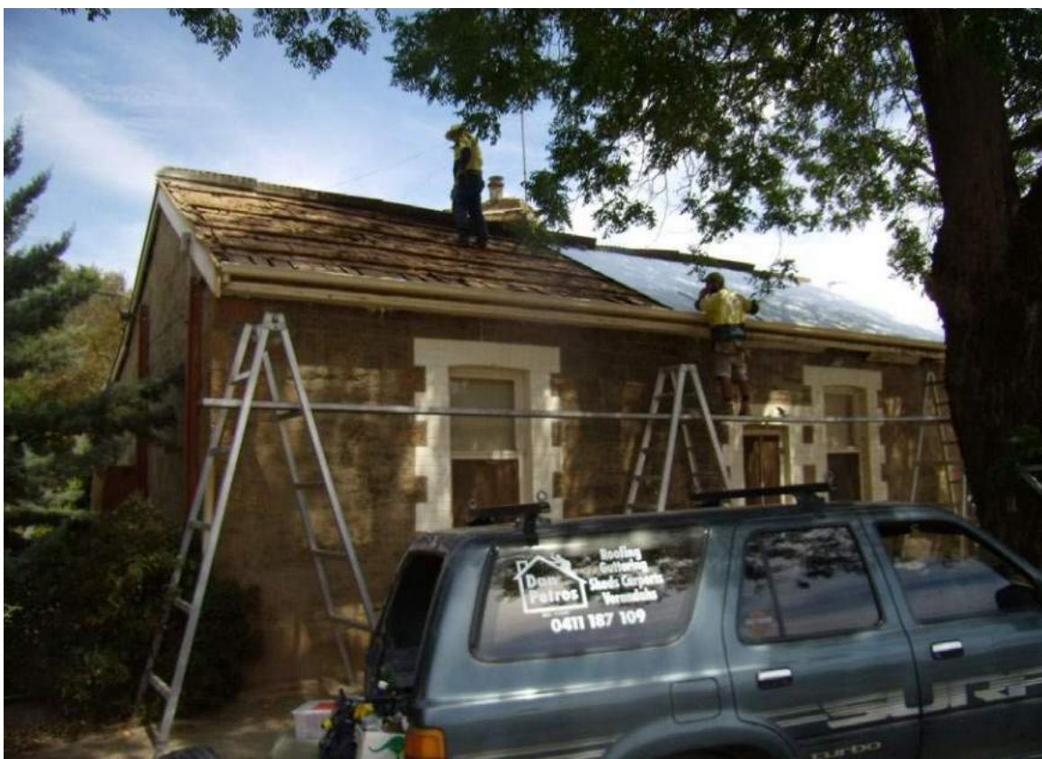
Original shingles revealed when re-roofing in February 2013. Source: Courtesy of the Burra History Group.
