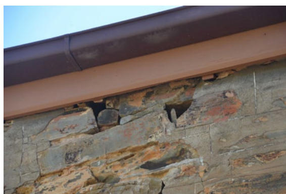
SAMA Storeman's Dwelling (SAHR 10049) – Deterioration of pointing to top of wall from earlier leaking gutter
