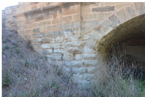
Mine Bridge (SAHR 10021) (Currently not mentioned in the National Heritage Values) – Severely decayed stonework due to penetrating damp from retained soil
