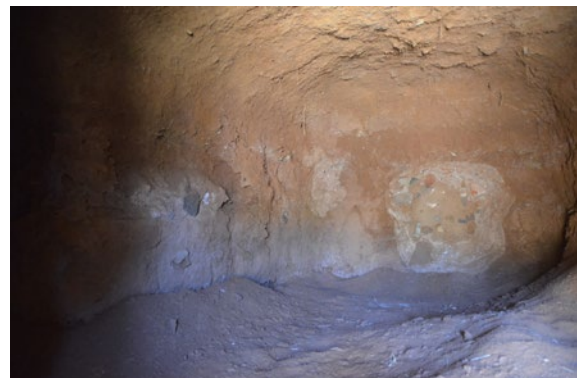
Miner's Dugouts (SAHR 10050) – Deterioration of clay surfaces
