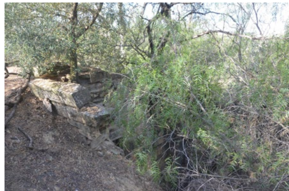
Structure of the former Waterwheel (Part SAHR 10970) – Vegetation growth within the masonry
