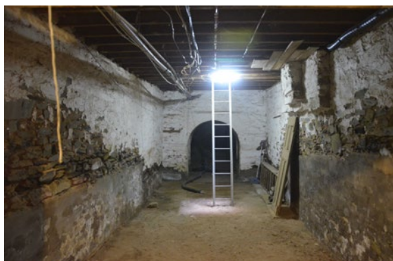
Burra Hotel Cellars (SAHR 10404) – Deterioration of mortar joints and stone due to soil backfill behind the walls
