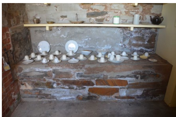
Burra Town Hall (SAHR 10403) – Salt efflorescence on internal wall surface caused by retained soil
