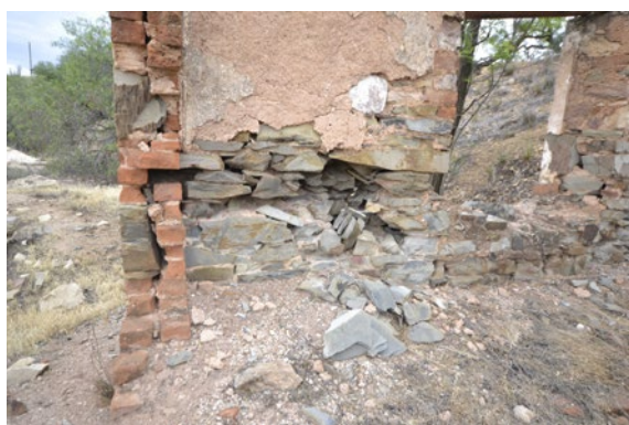
Mine Manager's Dwelling and Office (SAHR 10056) – Significant low level deterioration of stone and mortar threatening the remaining walls structural integrity
