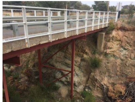
Julia Rd Bridge 2021 (prior to removal and infill)
