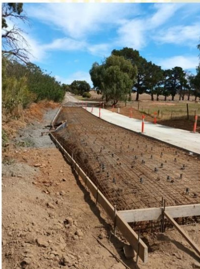
Mosey Rd Floodway – completed 2022
